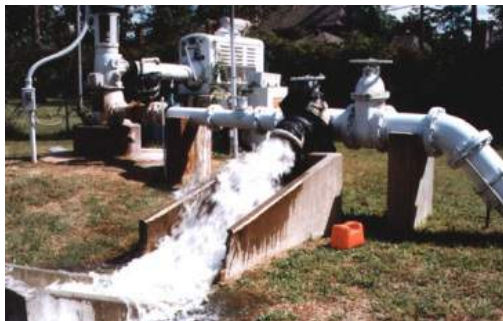
Figure 24 – Purging MUD Well in Northern Houston Area (Campbell, Campbell and Saribudak, 2004)
