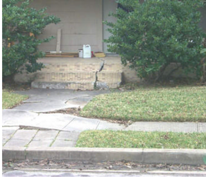
Figure 67 – GPR Profile 5: Hazard Street House (as of 2003) North to Right. Looking West (House Demolished in 2005 and Rebuilt)
